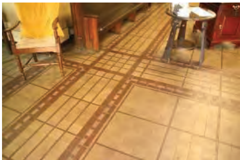
Figure 78: Floor tiling in the entry foyer (Source: 2013 CMP, p. 39)
