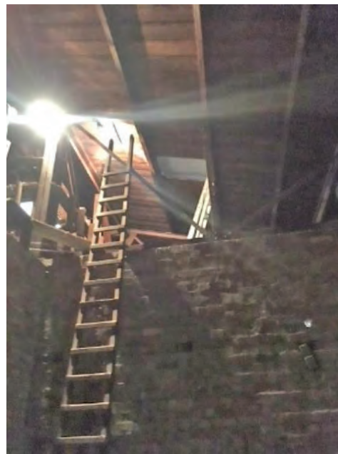
Figure 85: Roof space above the northern entry (Source: NBR SARCHITECTURE 2018)
