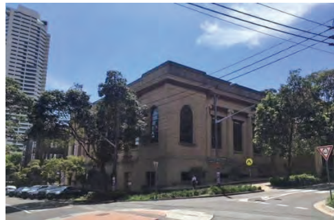
Figure 41: The south-west corner of the building, viewed from Liverpool Street (Source: NBR SARCHITECTURE 2018)
