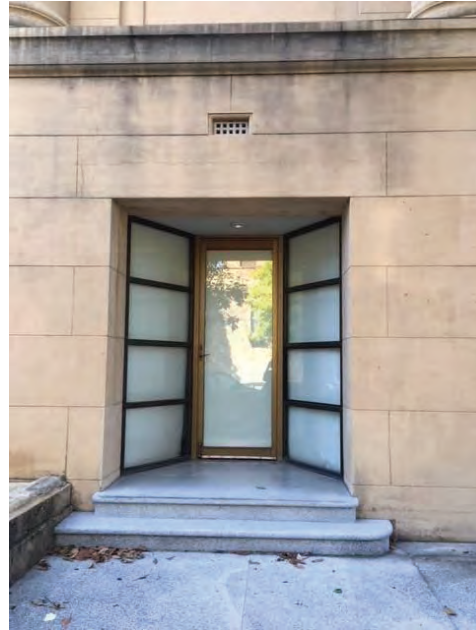
Figure 51: Lower ground level door on the western elevation (Source: NBR SARCHITECTURE 2018)
