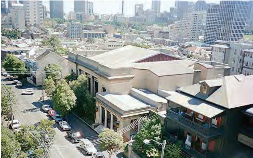
Figure 31: Bird's-eye view of the building (Source: 2013 CMP, p. 36).
