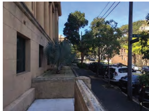
Figure 49: View of the western façade of the building, facing south down Forbes Street (Source: NBR SARCHITECTURE 2018)
