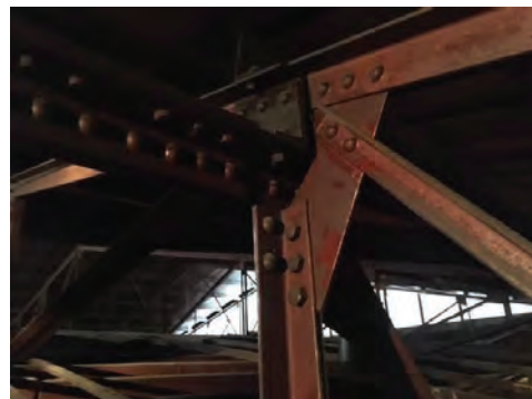
Figure 89: Steel roof trusses (Source: NBR SARCHITECTURE 2018)
