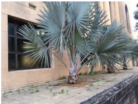
Figure 48: Pavers and planting behind the stone retaining wall on the western side of the building, above pavement level (Source: NBR SARCHITECTURE 2018)
