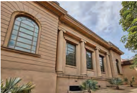
Figure 40: The south façade of the auditorium, fronting Liverpool Street (Source: Cornerstone 20181023_Shot_03_053.CR2)
