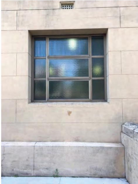
Figure 50: Lower ground level window on the western elevation (Source: NBR SARCHITECTURE 2018)
