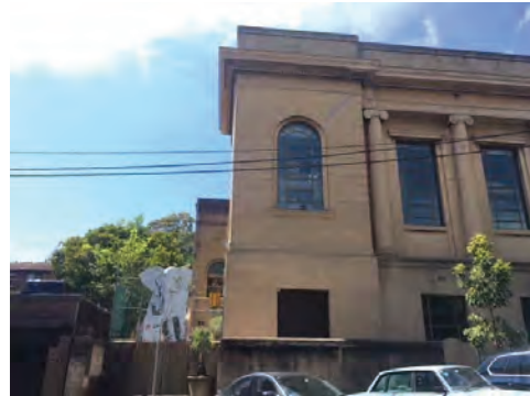
Figure 45: The north-west corner of the building, viewed from Forbes Street (Source: NBR SARCHITECTURE 2018)
