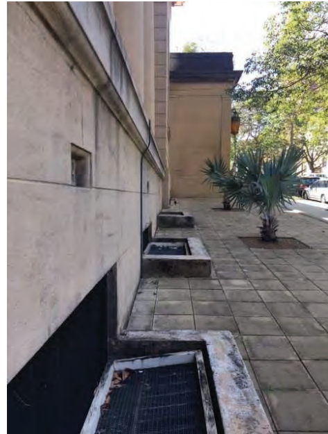
Figure 39: Light wells on the southern façade of the building (Source: NBR SARCHITECTURE 2018)
