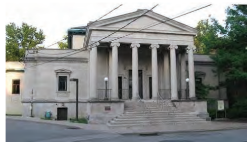
Figure 99: The former First Church of Christ Scientist, Pittsburgh, Pennsylvania, designed by S. Beman (Source: http://www.thefullwiki.org/List_of_former_Christian_Science_churches_societies_and_buildings )
