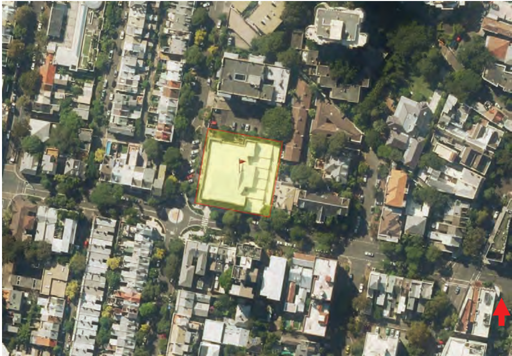
Figure 2: Aerial view of the subject site, outlined in red (Source: Sixmaps)
