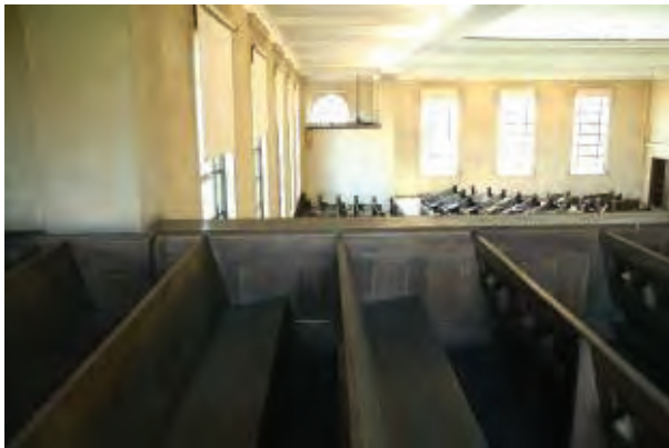
Figure 23: View of the choir gallery located above the corner stairs, prior to the recent additions (Source: GBA CMP 2013, p. 40)
